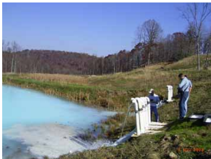
Figure 2: Passive treatment system.
