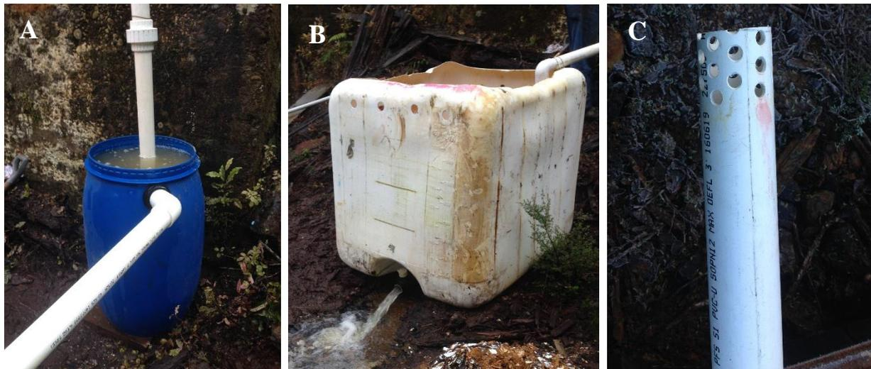
**Figure 4.** A. Image of diversion well with inlet piping AMD and an outlet allowing flow into settling pond. B. Image of IBC used as a settling pond. Water from well piped into top of settling pond, treated water outflow at base into Cannel Creek. C. Image of perforated 50 mm inlet pipe into diversion well.
